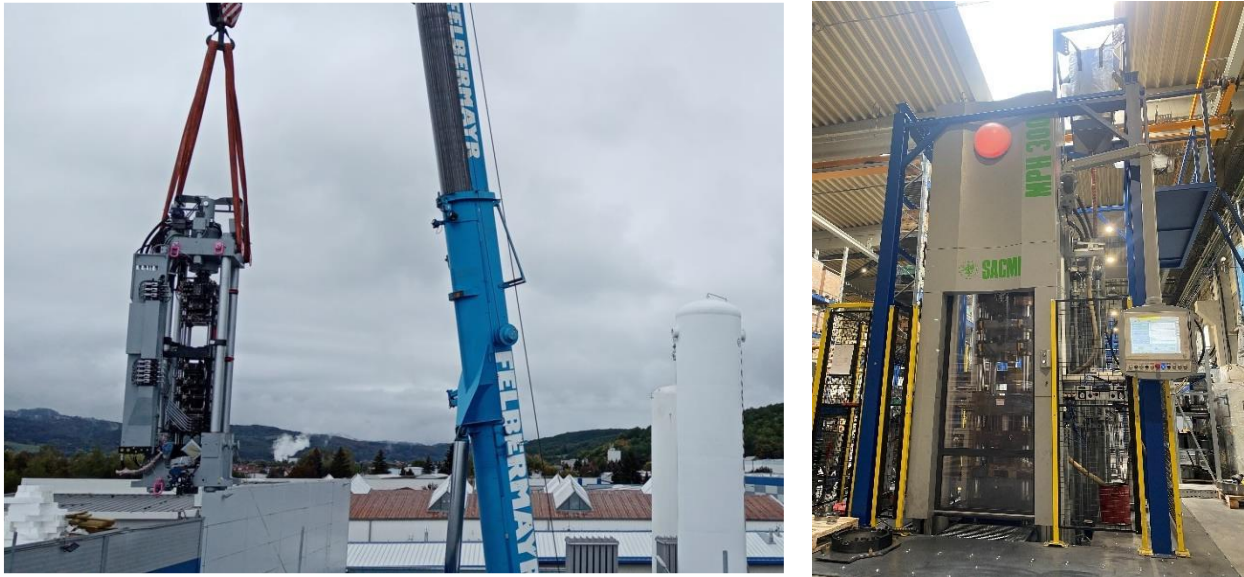
SACMI 300t press unloader (left), press after successful installation (right)
